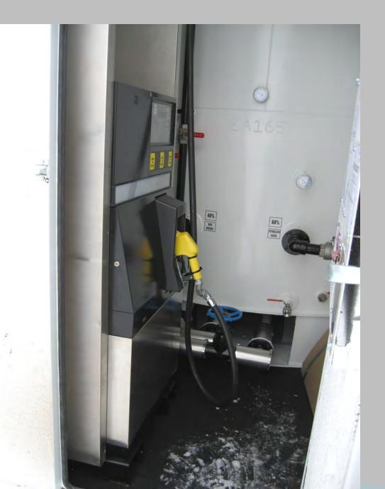
The blender dispensing system is able to mix three different blends of biodiesel, (B5,B20 and B100) on site.
